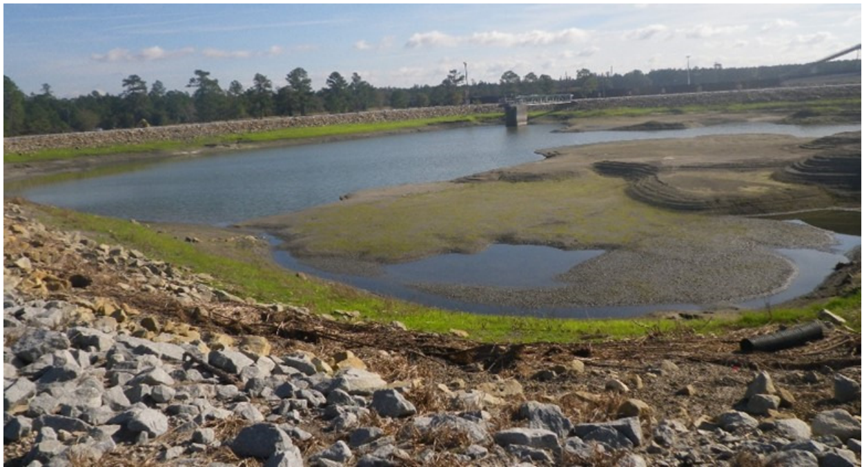
Figure 6. Variable CCR Surface in Ash Cell #2
