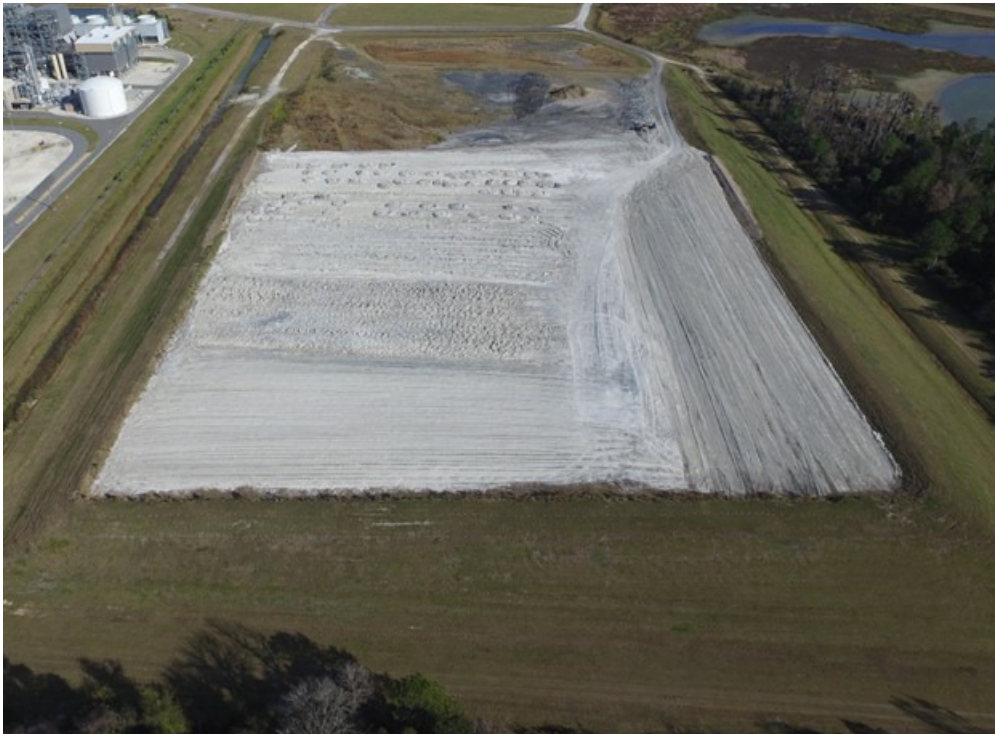
Figure 2. Aerial Image of CCR Landfill Facing East (IWCS 2016b)
